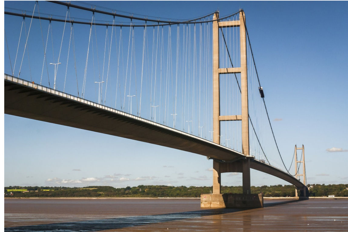
The Humber Bridge. Despite sluggish house prices in the region, people are still buying and selling well.
