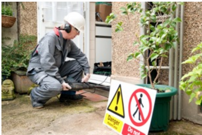
A property is treated for rising damp.
