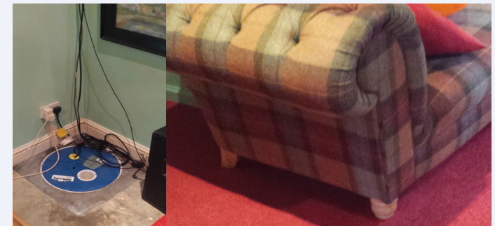
Figure 4 Sump pump (supplied from upper floor) and sofa on legs in the lounge
