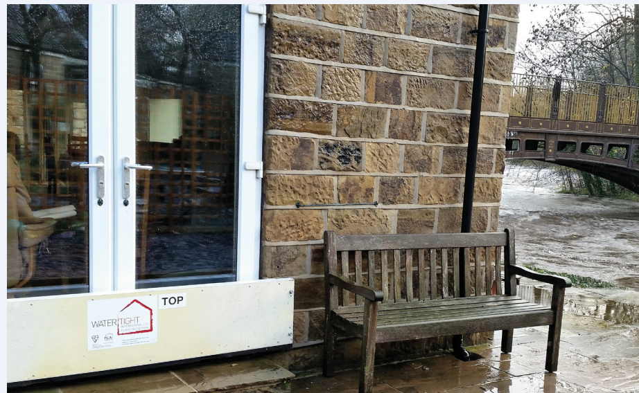
Figure 2 Although barriers were in place, the river had an unpleasant surprise in store
