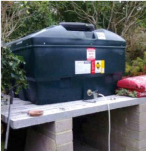
Figure 3 Fuel oil tank on raised plinth
