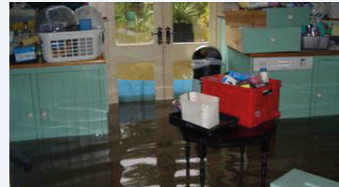
Figure 1 Kitchen during the flood
