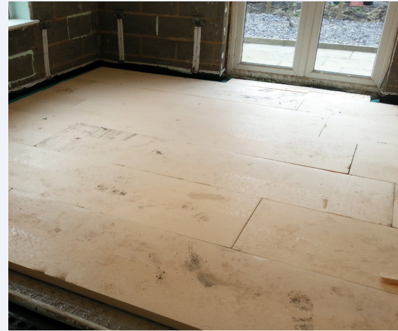
Figure 6 Closed cell (waterproof) insulation on the floor
